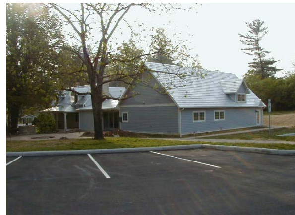
Left - a view of the Village Hall with the large meeting room on the right side of the picture. The large building is new construction.
